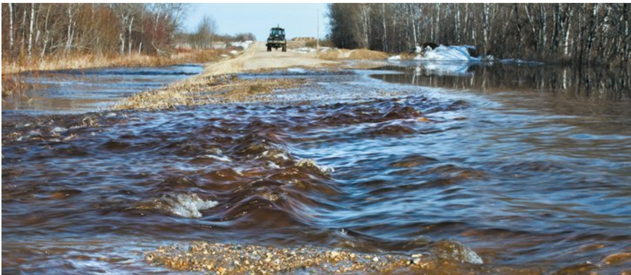
example of a draining wetland destroying a road
